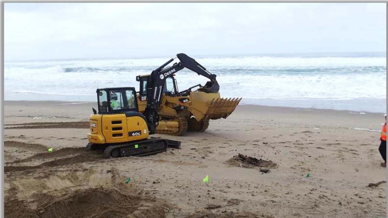
Sump material was loaded directly into the bucket of a tracked front-end loader which was then tracked back out along the beach and out the 7X Access Road. Sump material was dumped into haul trucks which then hauled the material to the M3 Stockpile Site.
