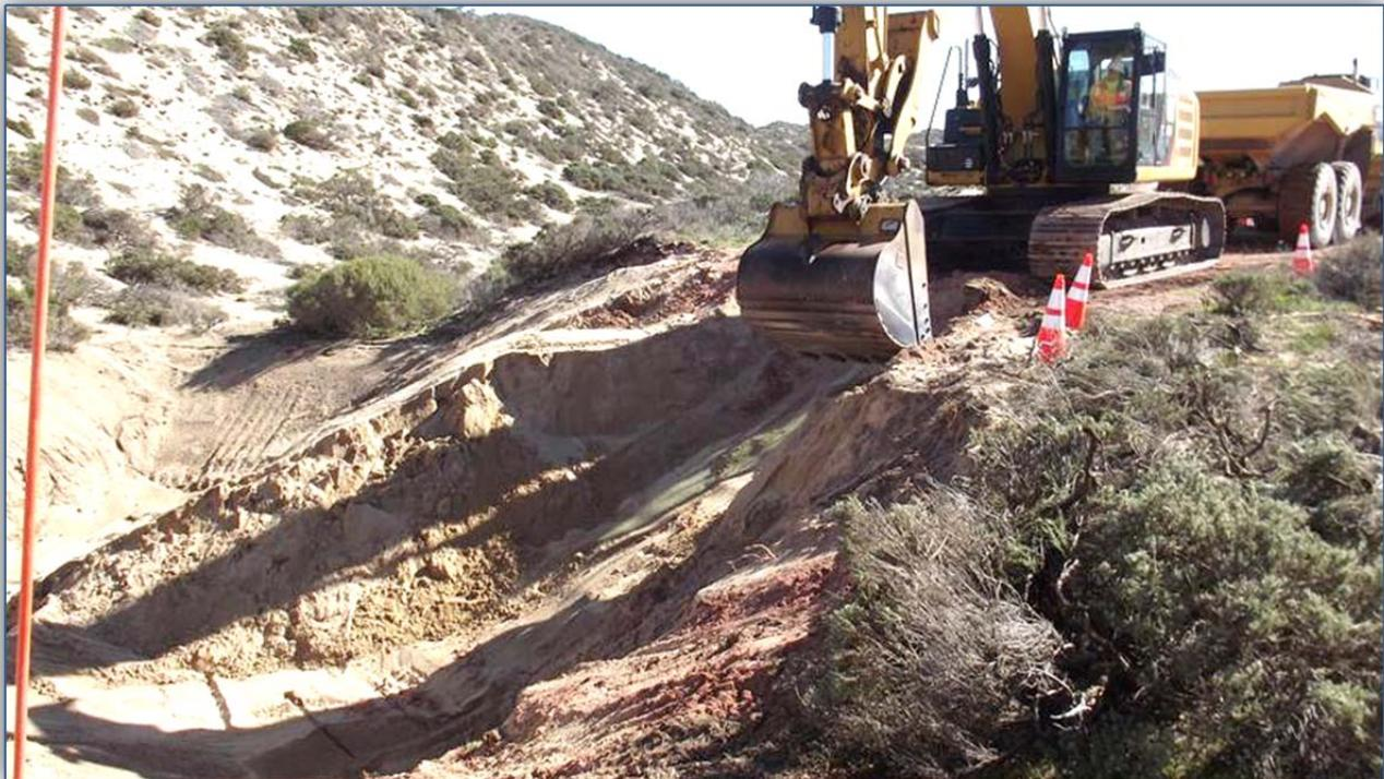
**J11 Pad Remediation Site:** area below the J11 Pad Site that contained diluent-affected material. Typical site activities include the removal of the sump material down slope of the pad, excavation of diluent-contaminated soil along the edge of the pad; and then future pad break-up after all excavations are completed.
