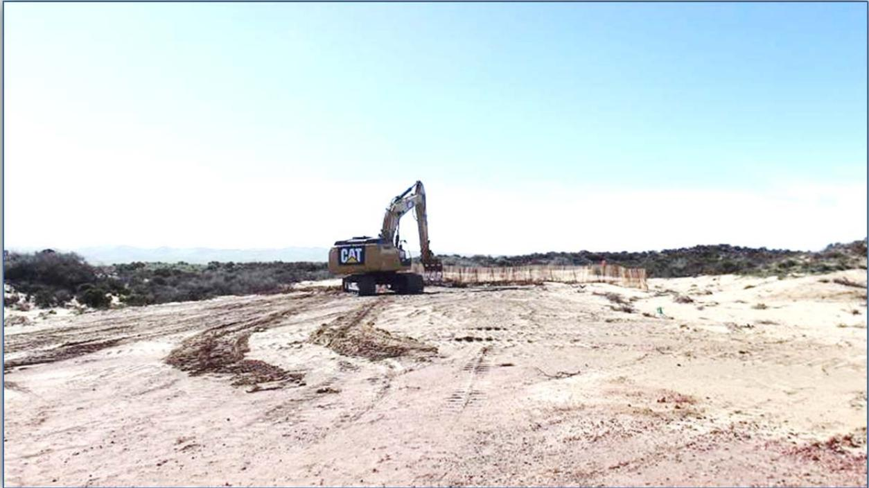
**M15 Sump Removal and Pad Treatment.** All of the sump material encountered in the excavation of this site was excavated; the remainder of the red rock Pad is currently being broken up with excavator and claw.
