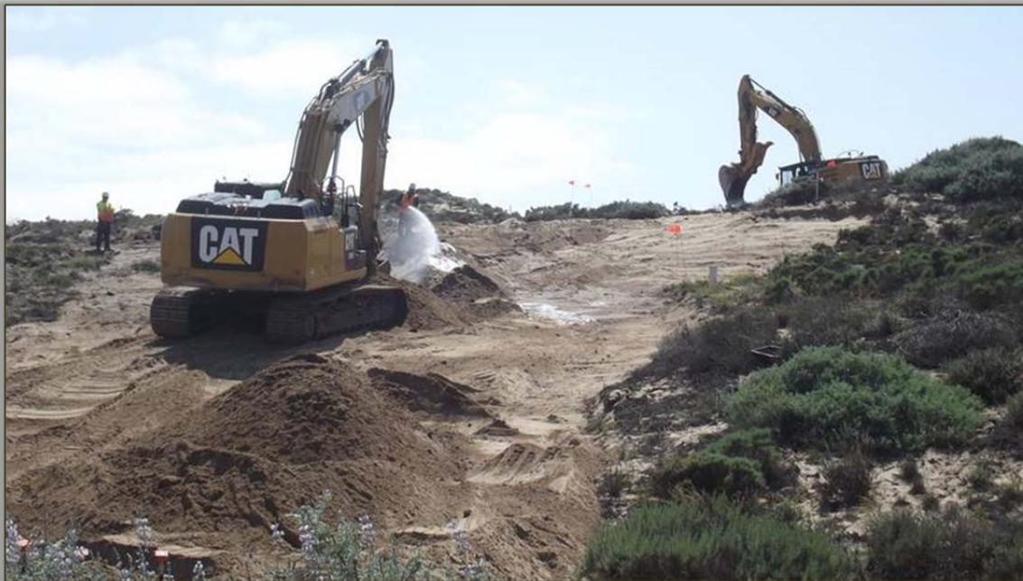
**I12 Excavation.** Two excavators have been used to excavate diluent-contaminated soil from this site. Note the use of water being sprayed on contaminated material which reduces dirty material being blown outside the controlled work area in windy conditions.
