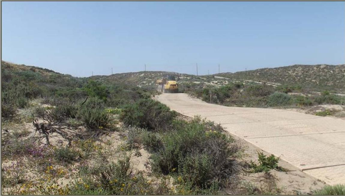
**Access Road to the I12 Excavation Site.** Entact has begun using plastic inter-locking mats to access more remote sites. Mats have, in general, reduced the total amount of required grading and reduced disturbances to subsurface roots which will likely improve restoration efforts.
